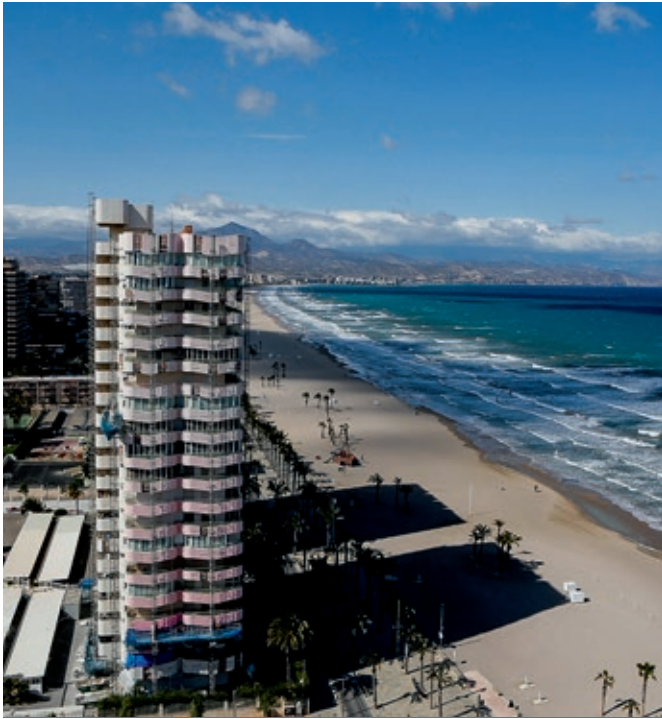
Buildings located in coastal areas
