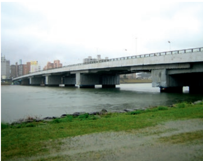
Tachibana Bridge, Japan
