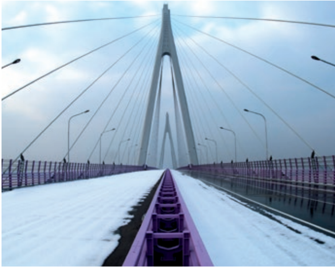
Hang Zhou Bay Bridge, People's Republic of China
