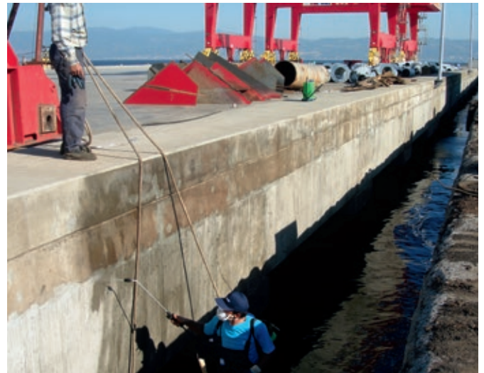
Yilport Jetty, Kocaeli, Turkey
